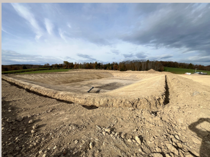
Site work complete with leak detection installed, awaiting liner installation.
