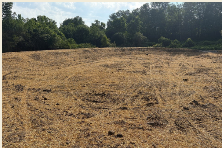
Project site post-construction, showing the newly constructed detention basin that will hold back stormwater during severe rain events and slow release it over a 24 hour period reducing damage to homes and roads below.
