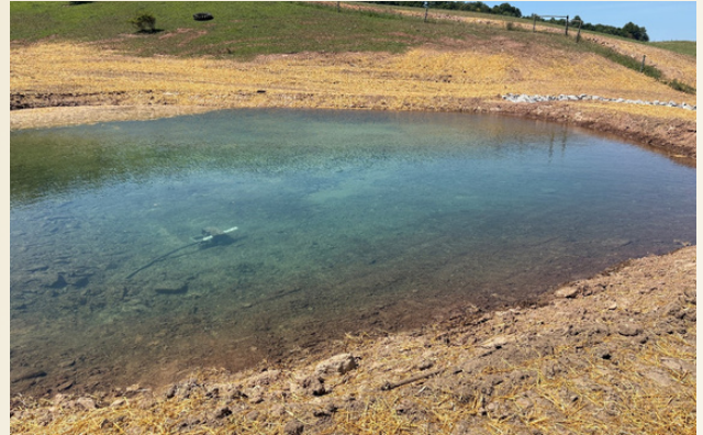
Pond after construction.
