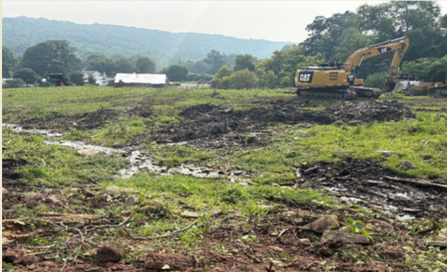
Watering pond before construction.
