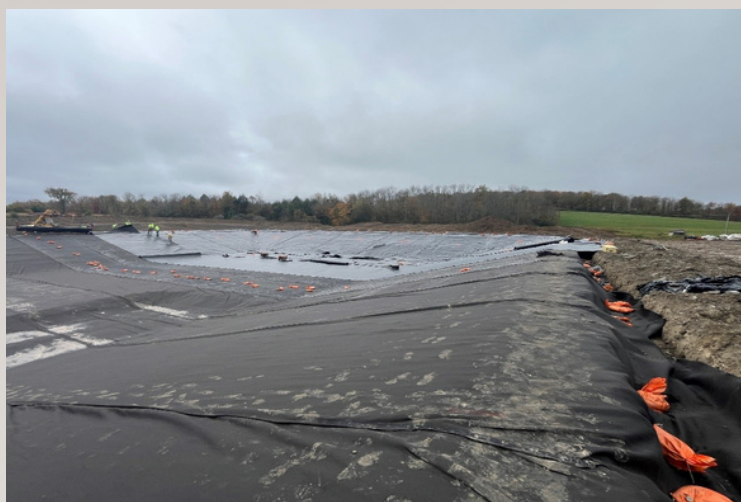
Polyethelene liner being installed.
