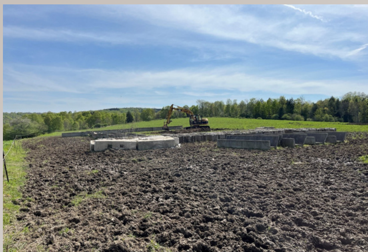
Site work under way.
