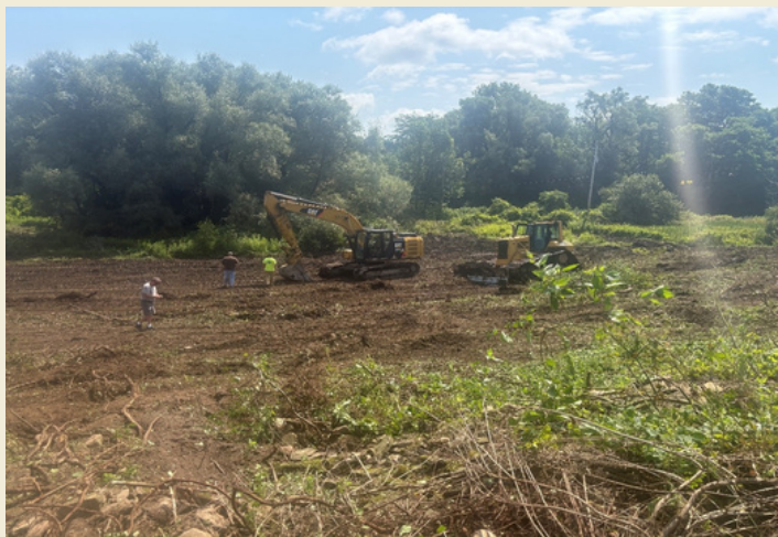
Site at start of construction.
