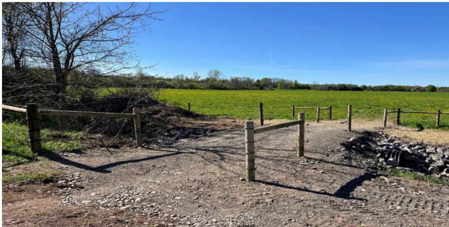
New fence and stream crossing after construction
