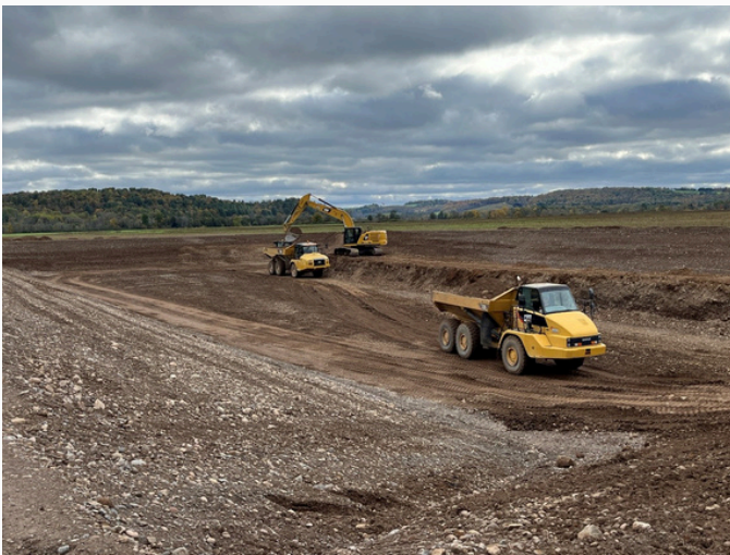
Site work underway
