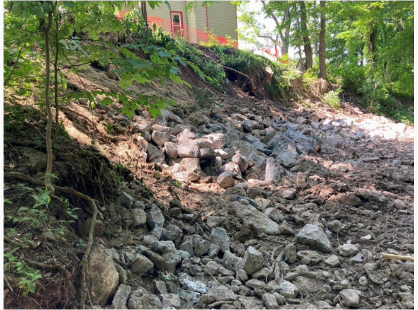
Project site post-construction, showing the installation of large riprap to eliminate the erosion and keep the stream channel from moving closer to the home
