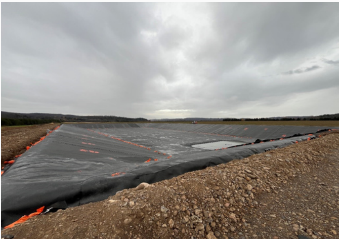
Polyethelene liner installed
