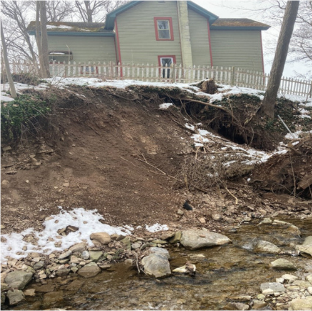
Site prior to bank stabilization
