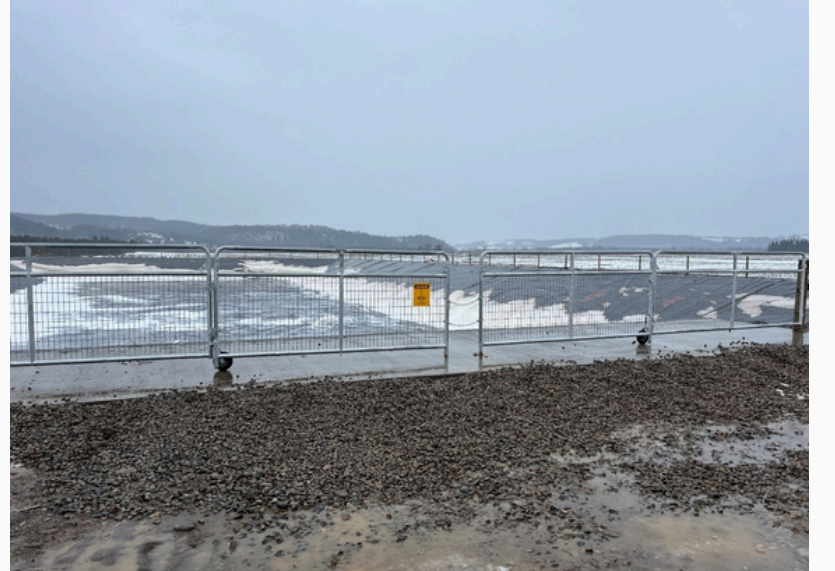
Project completed. Safety fence installed and ready for use.
