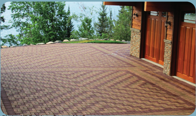
Photo: HT Builders, Permeable Pavers
