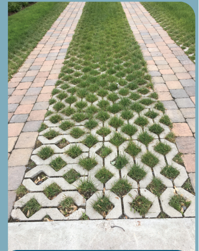
A Grass paver system allows water to soak into the ground.
