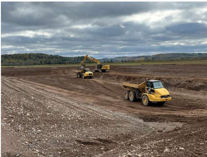
Site work underway
