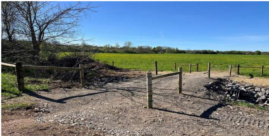
New fence and stream crossing after construction
