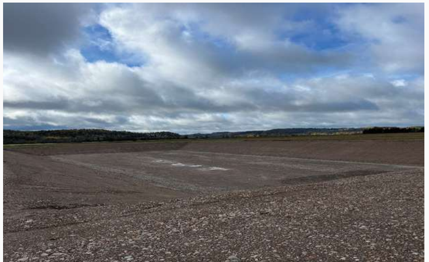
Site work complete with leak detection installed awaiting liner installation.
