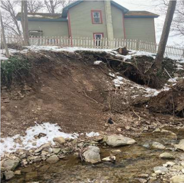
Site prior to bank stabilization
