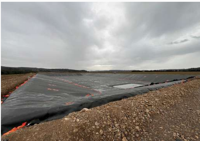
Polyethelene liner installed
